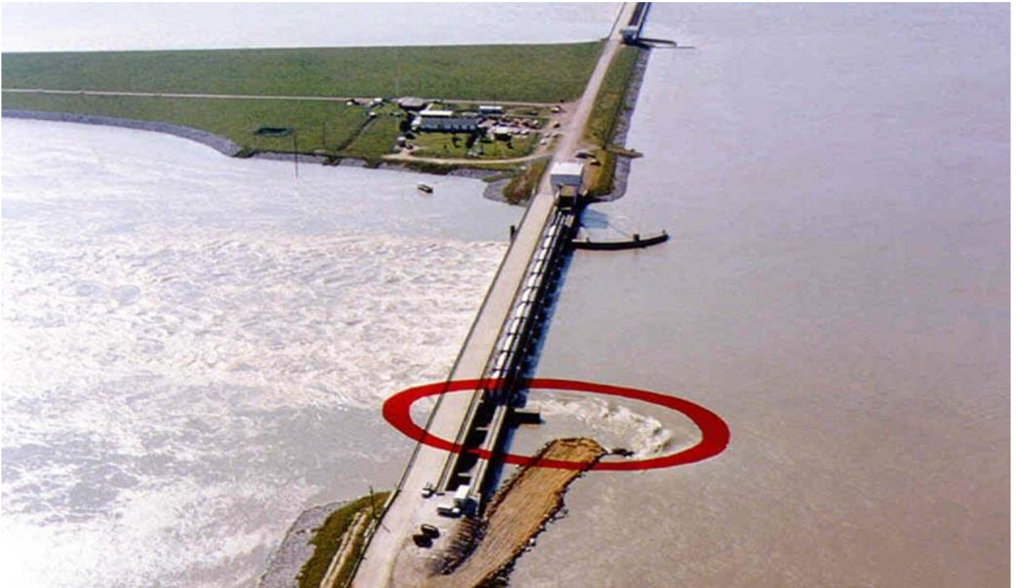
Figure 7: The Old River Control Structure's Low Sill Structure in April 1973. Scouring from a 1-in-40-year flood caused the 67-foot-long southern wing wall on the intake channel leading to the Mississippi River to collapse on April 14, and a large eddy (red circle) formed where the wall used to be. The eddy scoured out a 50-foot-deep football field-sized hole that undermined seven of the structure's 11 gates and nearly caused its failure. A ramp leading to the eddy was built, and an emergency stone replacement dike was built. Image credit: USACE . Special thanks to Dr. Jeff Masters.
