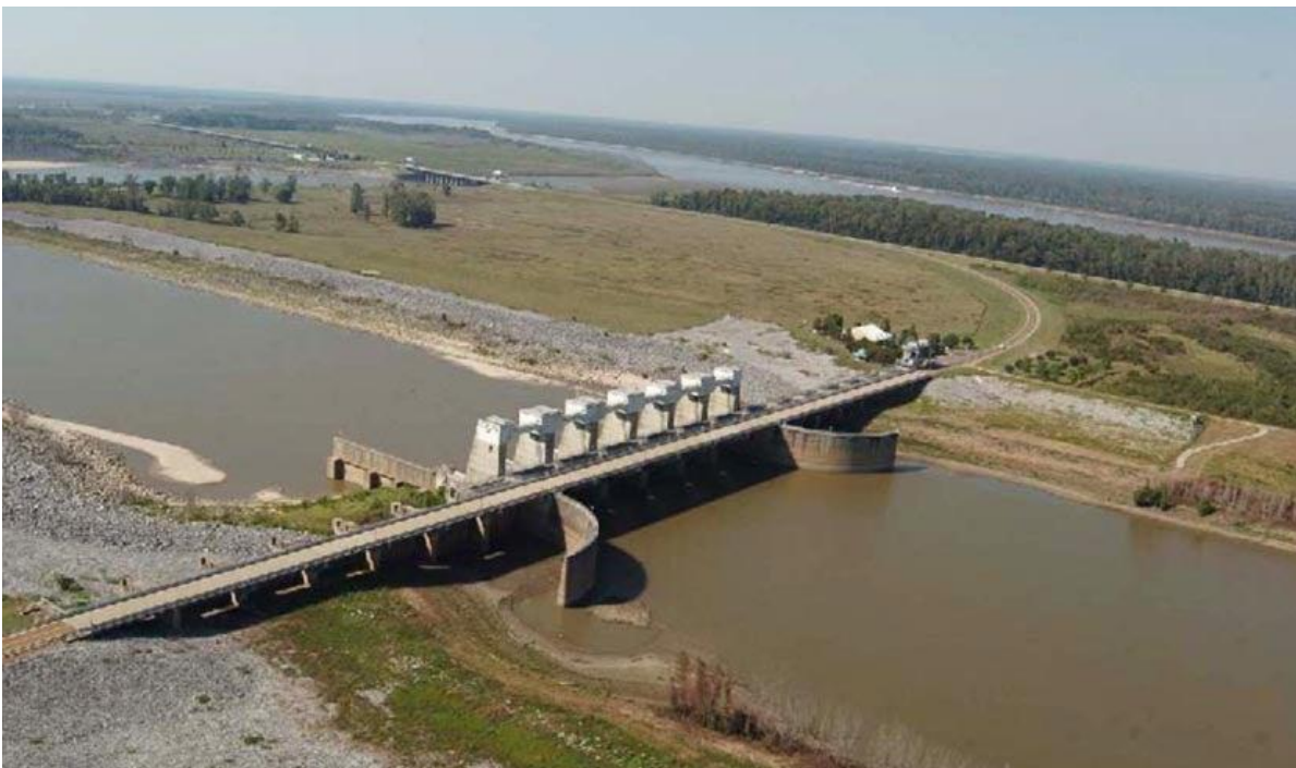
Figure 6: The Auxiliary Structure, the keystone of the $1 billion Old River Control Structure, which keeps the Mississippi River from changing channels. The main channel of the Mississippi River can be seen in the distance. Image credit: U.S. Army Corps of Engineers. Special thanks to Dr. Jeff Masters.
